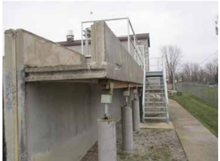
Aeration Influent Trough - Wall Deterioration and Temporary Supports - March 24, 2016
