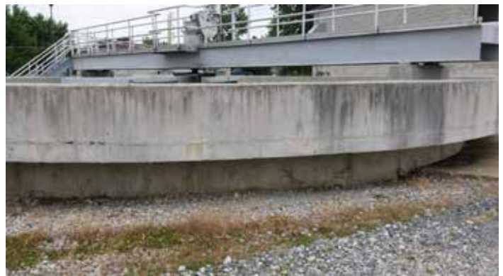
Clarifier Effluent Trough (Launder) - Wall Deterioration and Cracking - June 14, 2016
